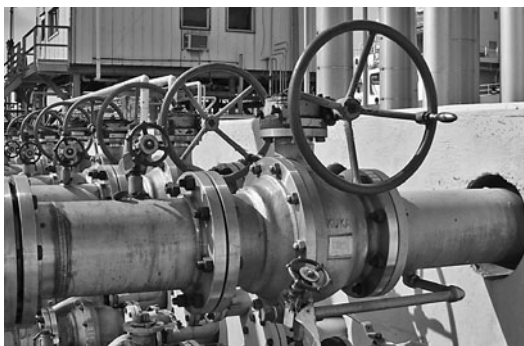
FIGURE 8.12 A bank of 8 in SS ball valves with manual right-angle gear operators with handwheels inside a chemical plant.
