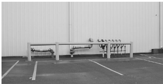
FIGURE 15.5 Pipe bollards and rails protect a service entrance near a parking area.
