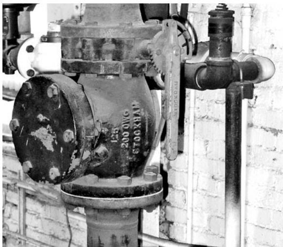
FIGURE 8.7 A cast iron swing check valve, 125 lb, with full-face gasket on upstream end, and lug-type butterfly valve downstream.
