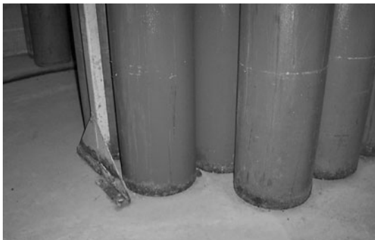
FIGURE 15.1 This structural steel storage rack and gas tanks for a fire protection system were exposed to a saltwater flood, but were left in the mud for a period of several weeks. The portions embedded in the wet mud began to corrode.
