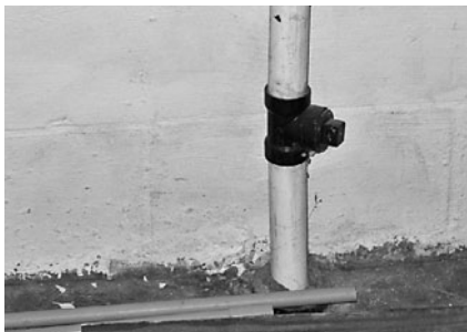
FIGURE 6.8 Plumbing code violation. Solvent welded joint (PVC welded to ABS test plug fitting).
