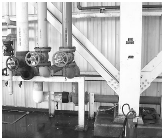
FIGURE 8.32 A cross connection between a potable water line and a fire protection system. The second riser from the left is potable water from the city supply; the third riser supplies the fire protection system. If the potable water pressure drops, nothing prevents the stagnant and iron-laden fire protection water from entering the potable supply.
